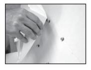
7. Line up the screw heads with the holes on the repositional base, and slide the unit down slightly until the screw heads are securely fastened to the repositional base.
